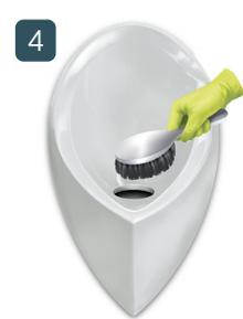
Clean the inside of the waste trap and urinal opening with a brush.
